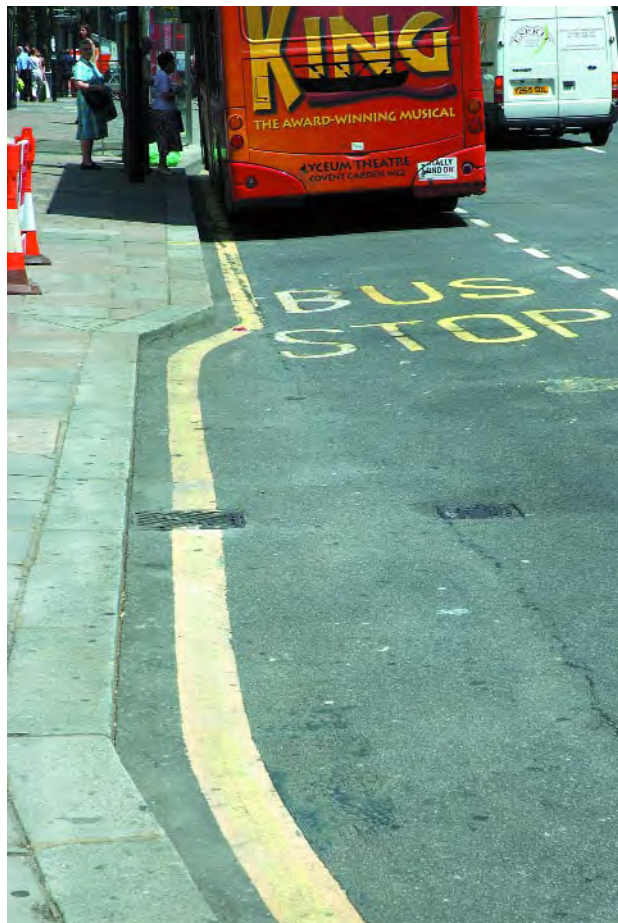
Partial build-out within bus bay
